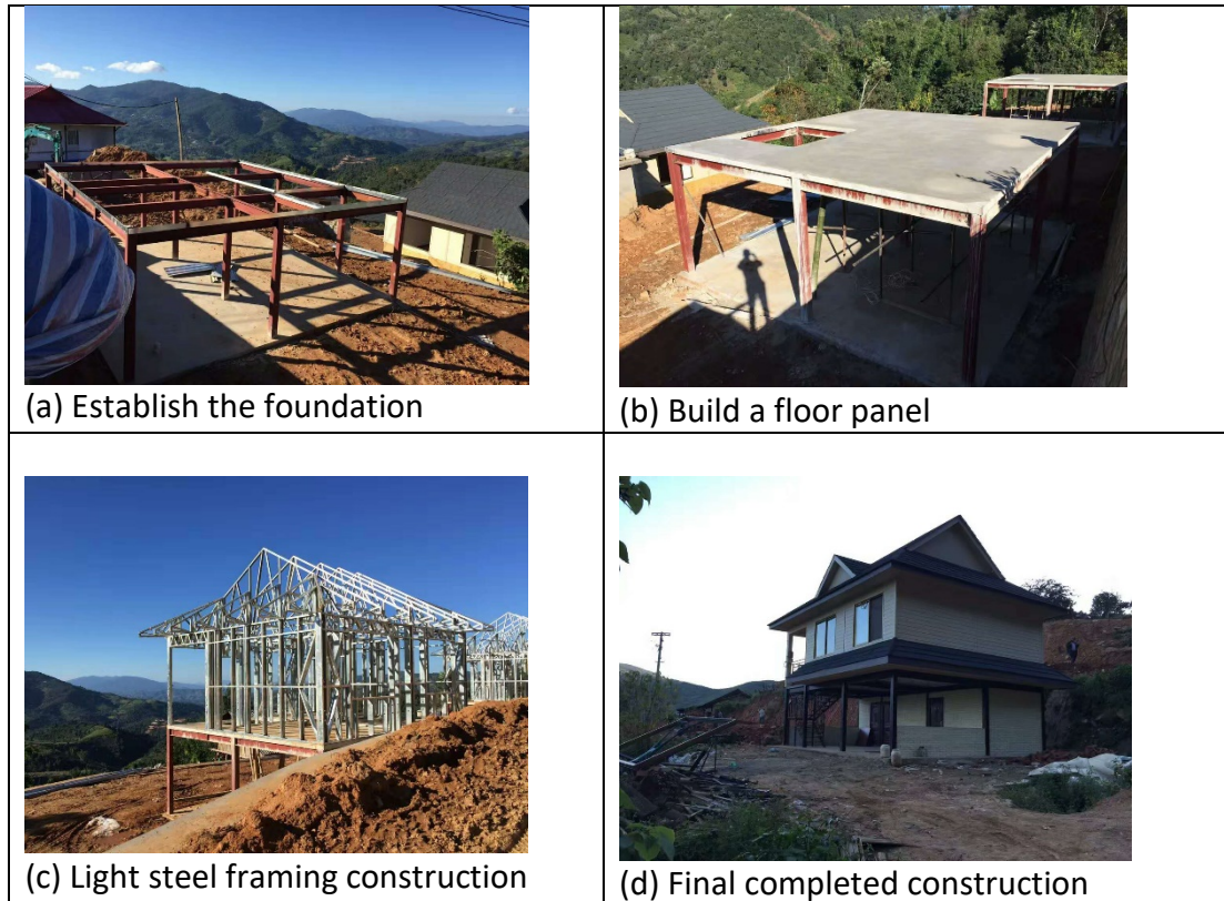
Fig. 3. Building process (source: photo by authors)
