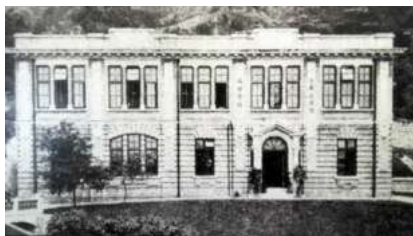
(a) A photo of a demolished building
