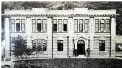
(a) A photo of a demolished building
