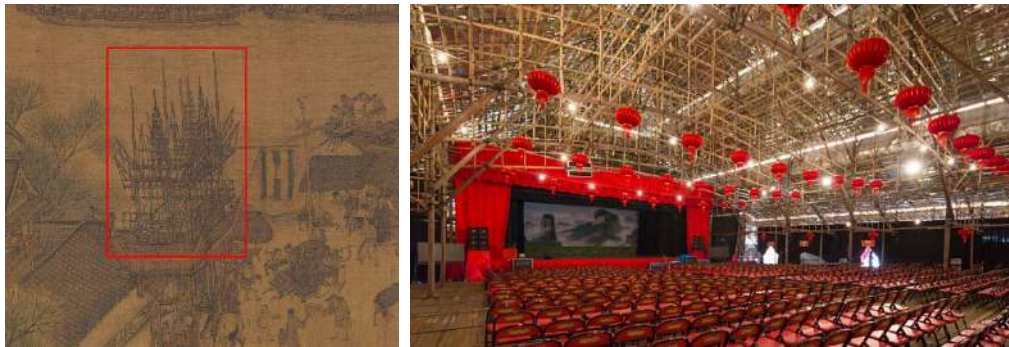
Figure 1 Traditional bamboo temporary structure. (a) Bamboo scaffolding-like structure in “Along the River During the Qingming Festival” (b) Temporary bamboo opera theatre
