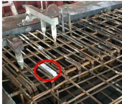
(g) RFID installation
