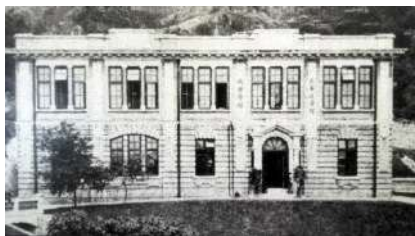
(a) A photo of a demolished building
